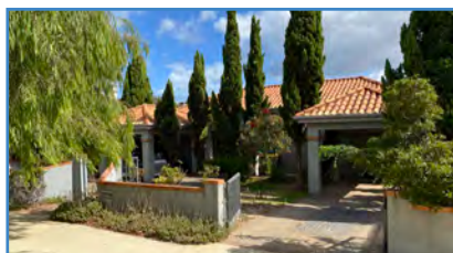
Existing suburban residential development fronting Shenton Road
