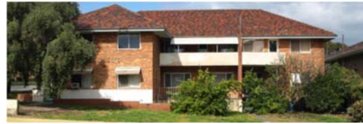
Condition of buildings
