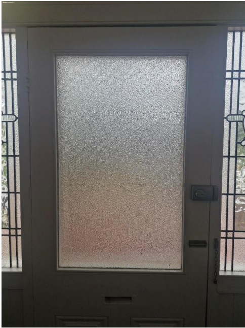
Image 4: 73 Shenton Road, current Glazing (July 2025)
