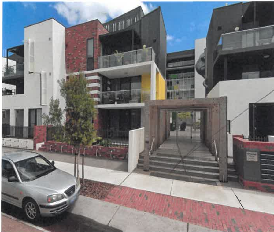
4-6 storey residential development with human scale and townhouse character fronting the public realm
