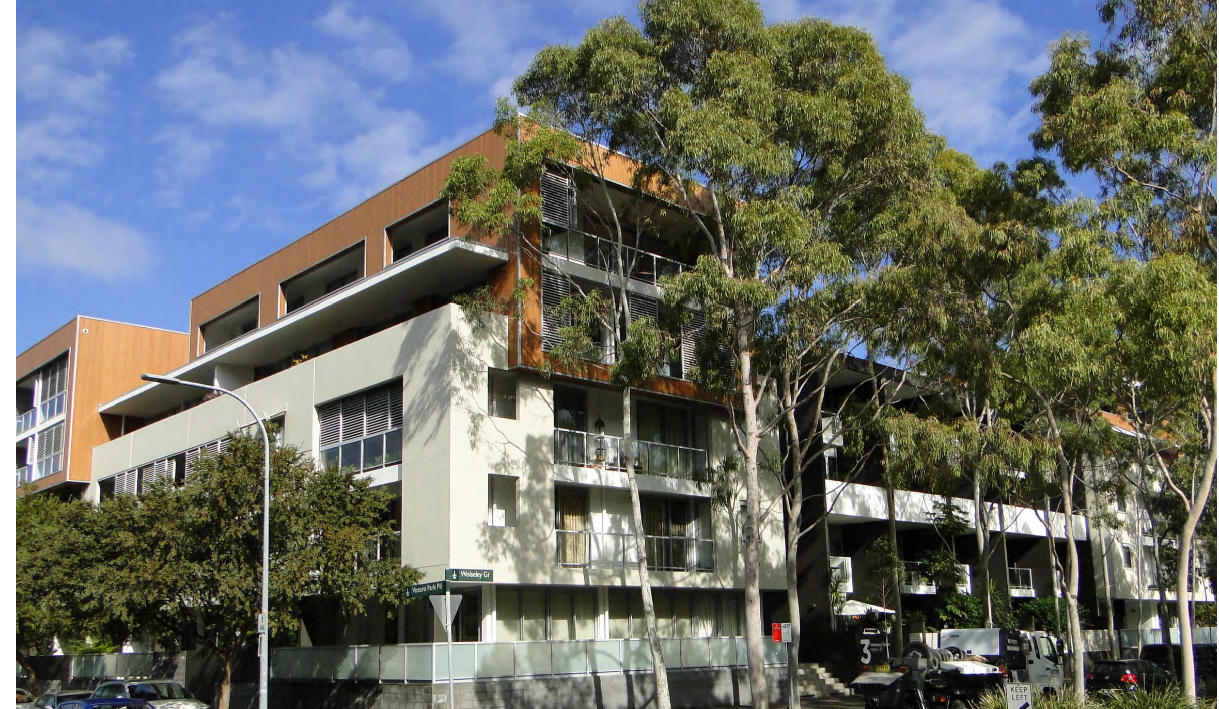
5 storey residential development retaining mature trees and 'human scale' to street
