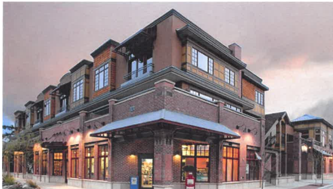
3 storey mixed use development with upper-level set back above heritage ground floor shops
