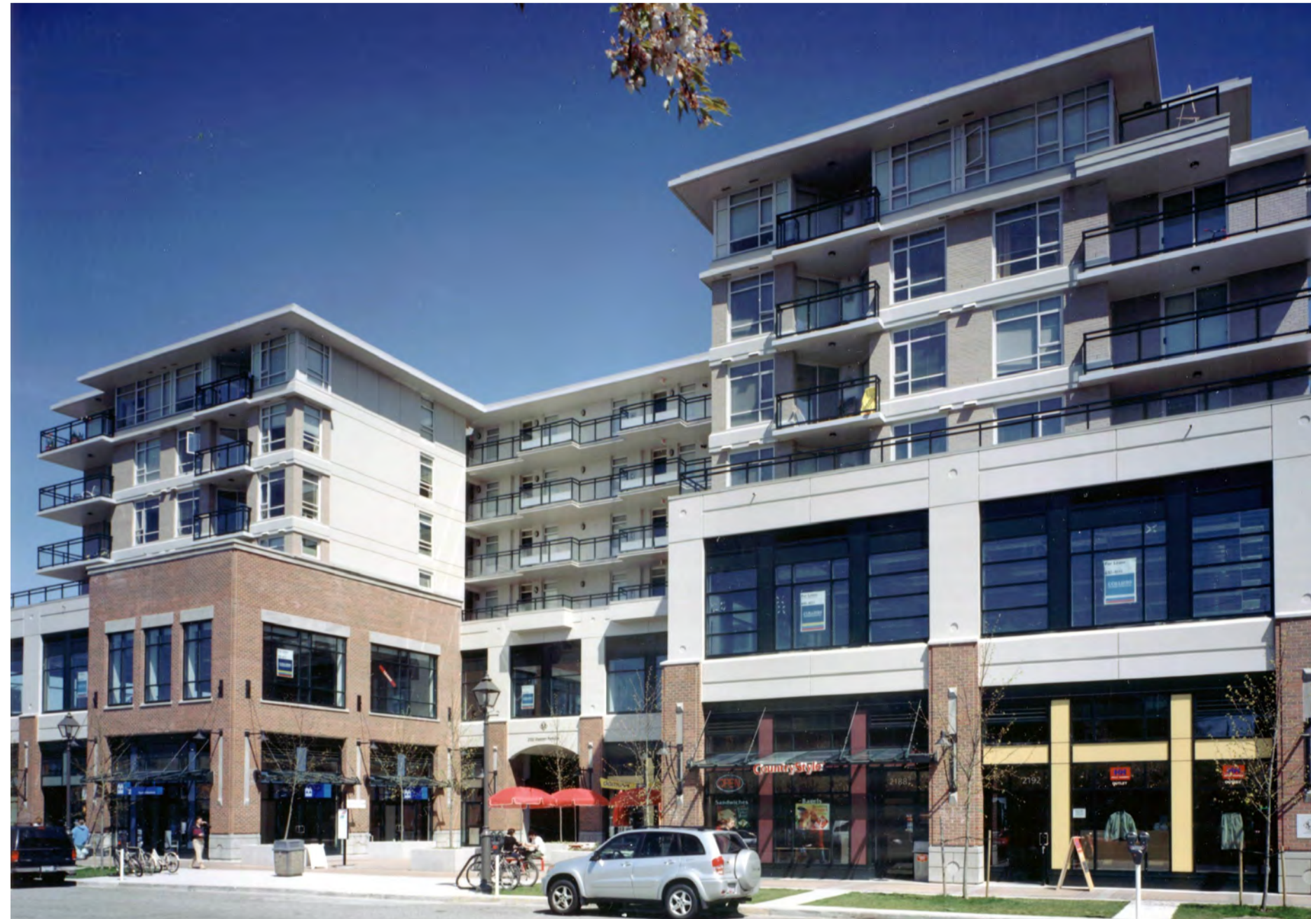
6 storey mixed use development with upper-level setbacks
