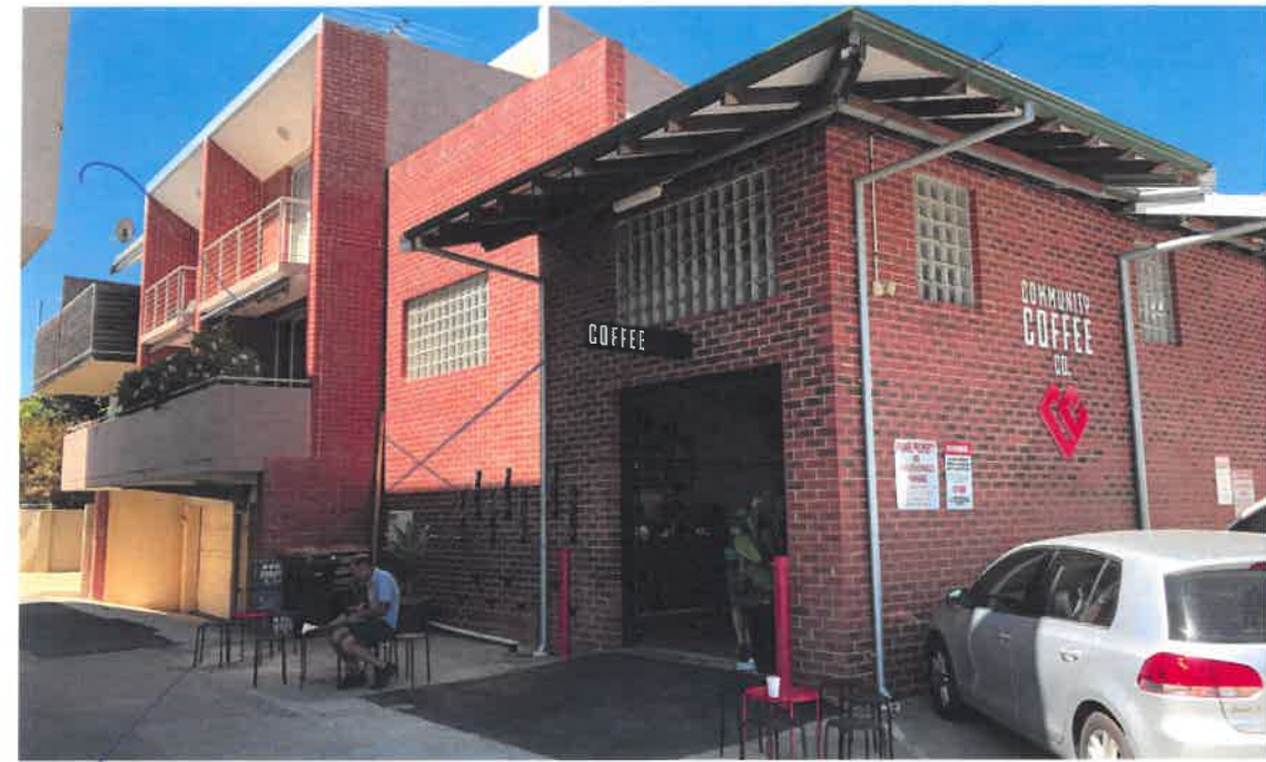
Repurposed heritage café with new 3 storey residential development
