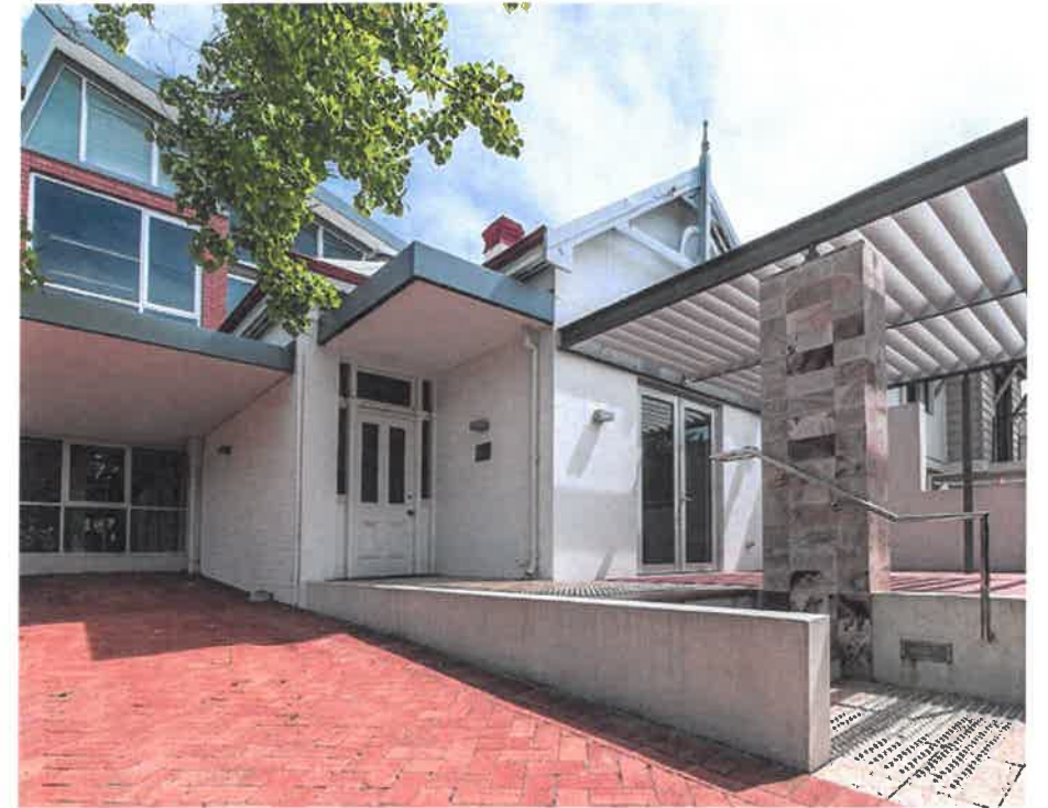
Former heritage home facade retained with new office extension behind
