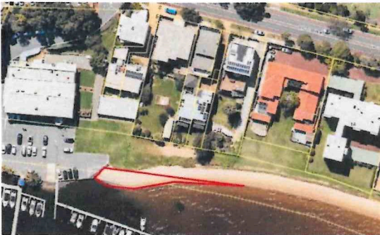
Sand to be removed from East of Claremont Yacht Club.
